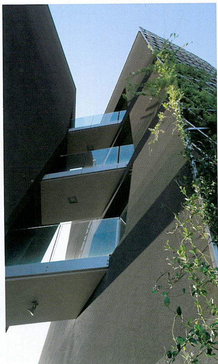
Detail of a façades section. Below and opposite page, views of the balconies connecting the two wings of the building and section across the stairways system with plants set at various heights.
